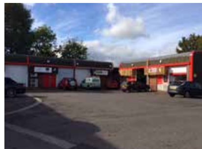
Farnham Farnham Business Centre Small business unit scheme managed for owner
