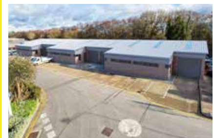
Units A-F Barwell Chessington 2338 - 14040 sq ft Fully refurbished To Let for Aviva
